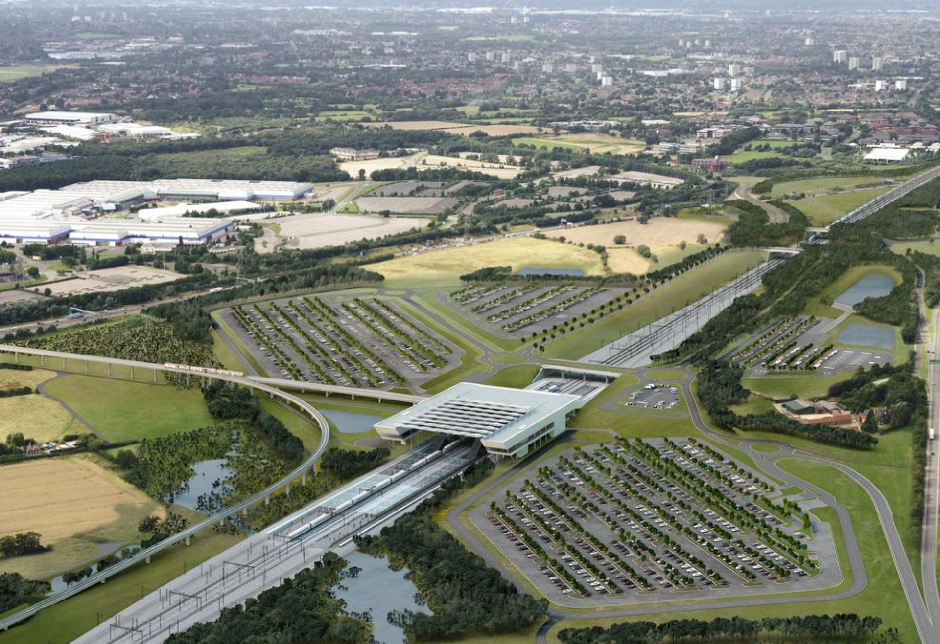
Birmingham Interchange station
